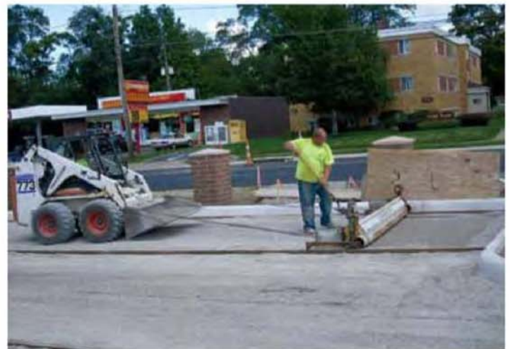
Figure 2. After compacting the No. 57 stone, No. 8 stone for the bedding layer is screeded smooth to receive the permeable pavers.
