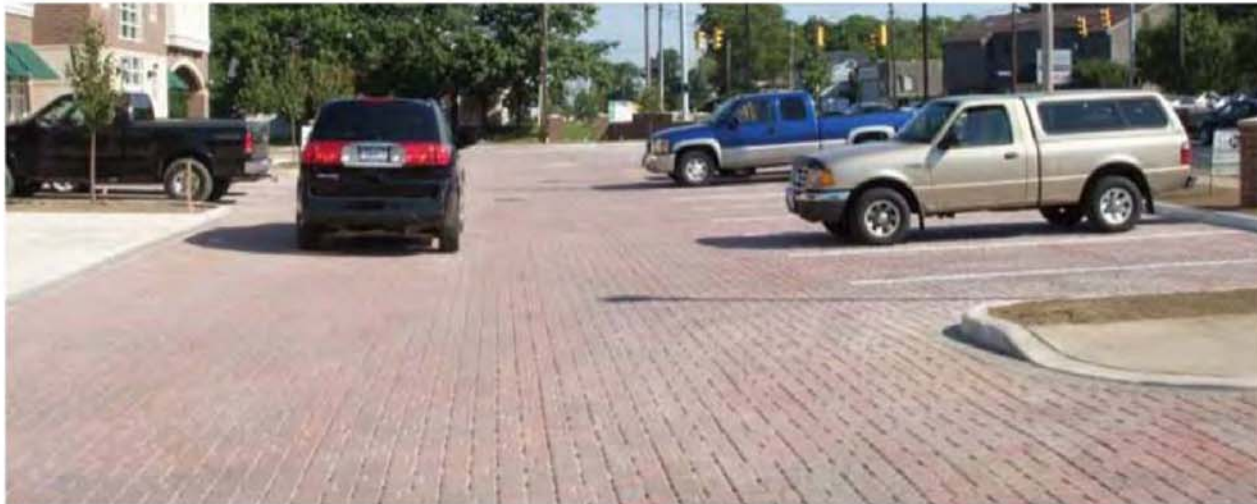
Center Street Village in Mentor, Ohio used over 140,000 sf (14,000 m 2 ) of old-style permeable interlocking concrete pavement to simulate stone paving in a mixed use project.
