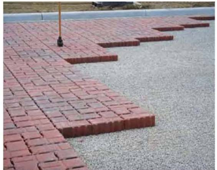
Figure 4. The offset rectangular laying pattern of the permeable paver clusters enables greater interlock.
